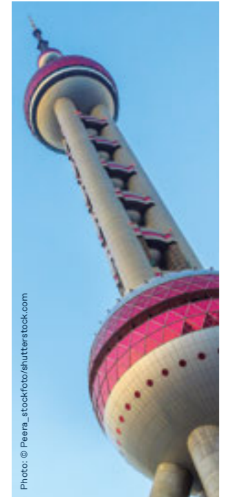
● Shanghai Pearl Tower, China
