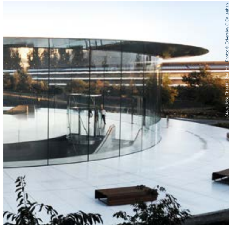
• Steve Jobs Theater Pavilion, Cupertino, USA
